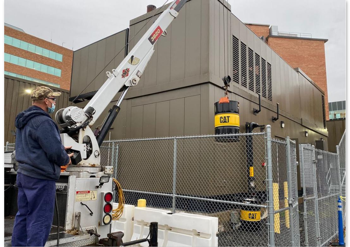
Installing a G3516H 2MW CHP plant
