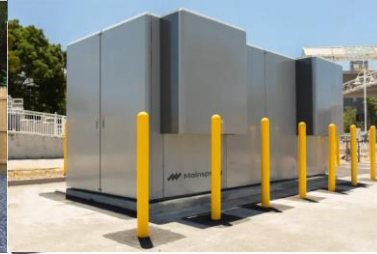
Fuel Cell CHP Units
